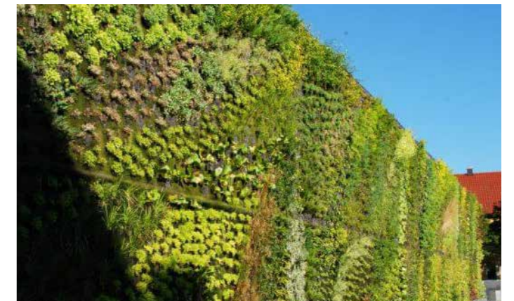
A green backdrop will provide texture, interest, greenery and will help screen the store yard behind.
