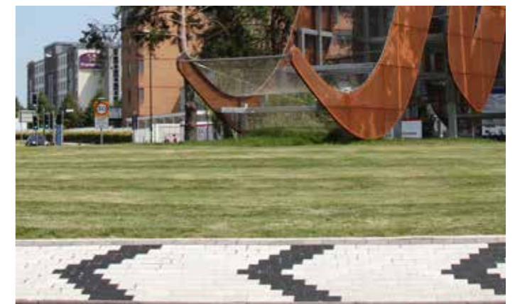
Changes the edges of the roundabout to chevron will minimise the need for signage and will make Gateway 1 look and feel the same as Gateway 3.
