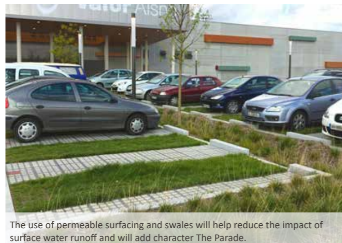
Materials to be consistent with other recent improvements in Manor Royal.
