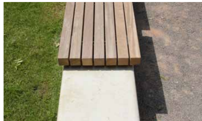
Seating walls help define the edge of the micropark and also provide incidental seating. Timber seating tops provide more formal places to sit.
